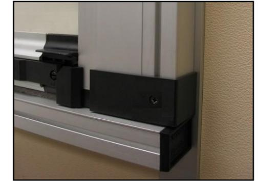
Fitted sill with correctly set inner and outer channels
